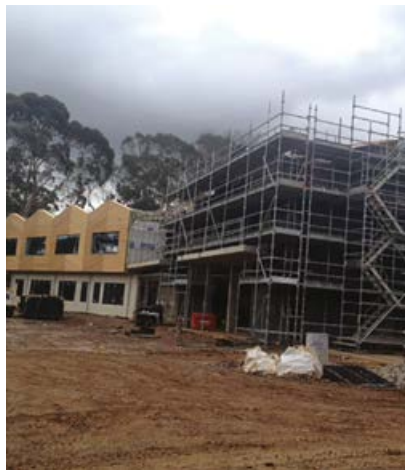
Belgrave Hub building in progress.
